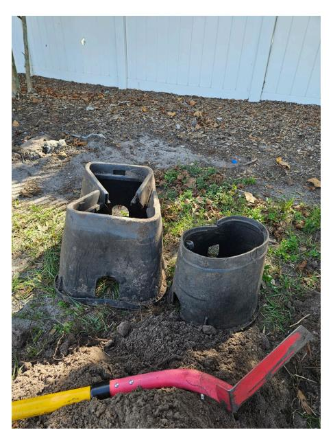
Damaged valve boxes along Balm, east of Ayersworth, need to be replaced as soon as possible since the open area does represent a tripping hazard. The area has been identified with yellow caution tape, but this is temporary at best.
